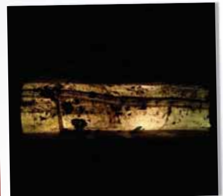
LIGHT TRAIN CURING LINER
