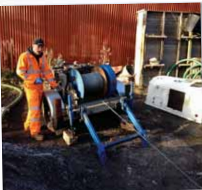
LINER BEING WINCHED IN
