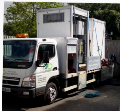
UV LINING RIG
