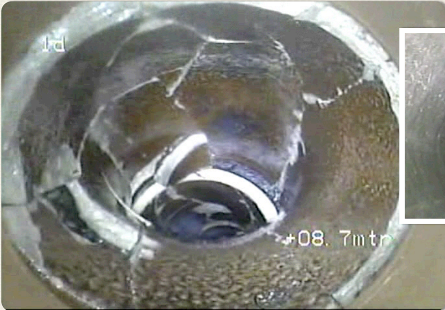
LEFT; BEFORE ROBOTIC CUTTING AND UV LINING.
